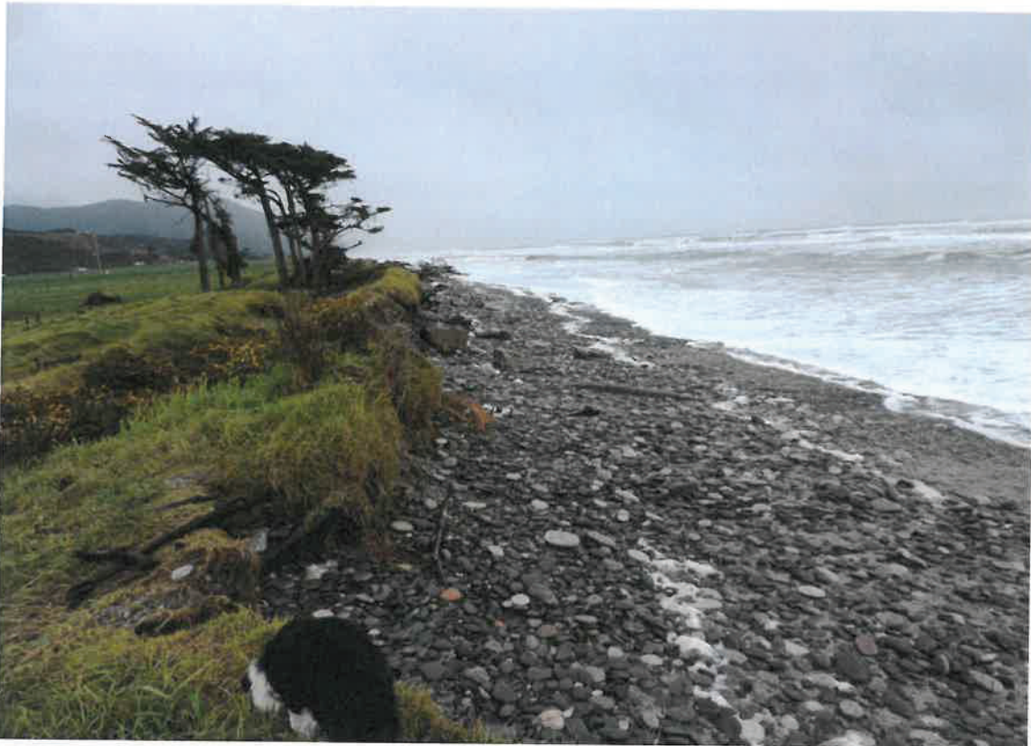
Photo 1: Showing erosion of the sacrificial bund - looking north.
