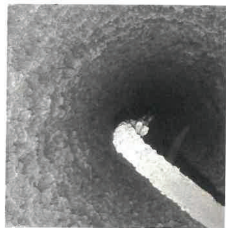
Light grey dust, approx. 5-8mm evenly spread on lower flue wall, 3 September
