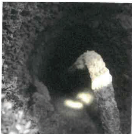
Wood-coal soot, less than ¼ the distance between the lower flue wall and the bottom of the electrode, grey/black colour, 27 June
