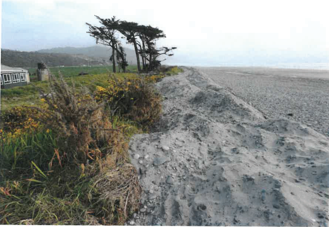
Photo 2: Re-constructed sacrificial bund
